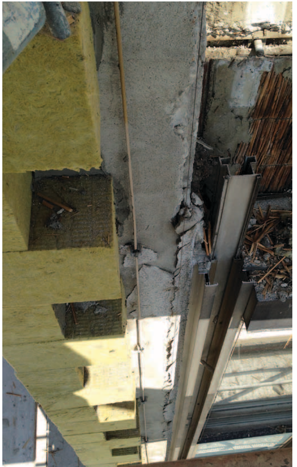
Schüco AWS/ADS 70.HI Tiptronic ASS 50 Facade FW 50+ Ruukki sandwich panel 200 mm Sun Breakers
